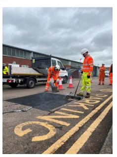
Following a test period the council and its public realm contractor, Balfour Beatty are continuing with the use of Mastic Asphalt to help improve the management of defects on the county's roads.
